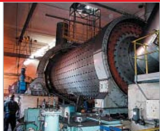
Pneumatic mill Ø 3.4 x 7 m for petcoke grinding
