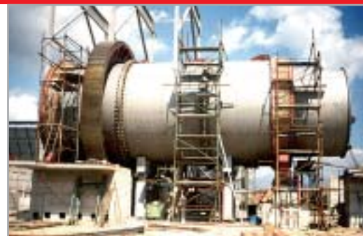
Assembly of a raw mill \varnothing 5.4 x 11 m with pre-drying chamber
