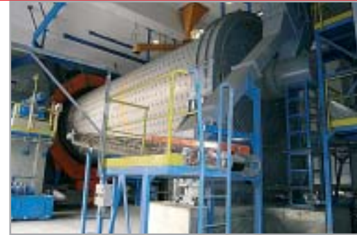
Cement grinding with a Ø 4.0 x 13.75 m mill seated on shoe-type bearings
